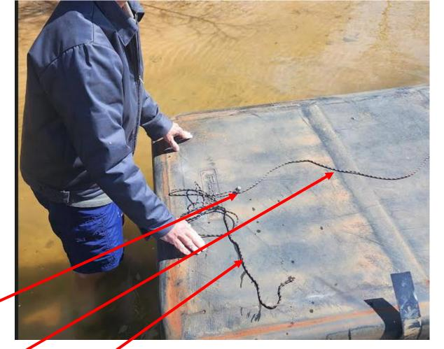
Leave about ½ inch of the bolt/screw exposed, the remainder being firmly hammered into the dock float.
